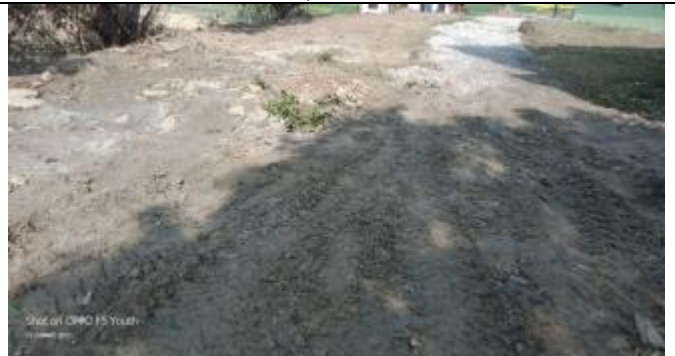
Office Building construction area (150 sqm) within Municipality compound
